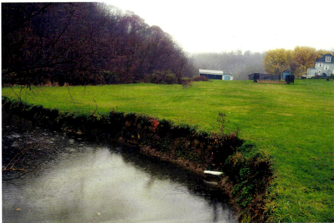
Figure 19. Streamside pastures along Enlow Fork (top is upstream, bottom is downstream) in a reach where drains have been constructed to prevent wetland development following subsidence from longwall mining, Greene County. The streambed here has been converted from riffle to pool habitat, with consequent reduction in fish and other aquatic biota.
