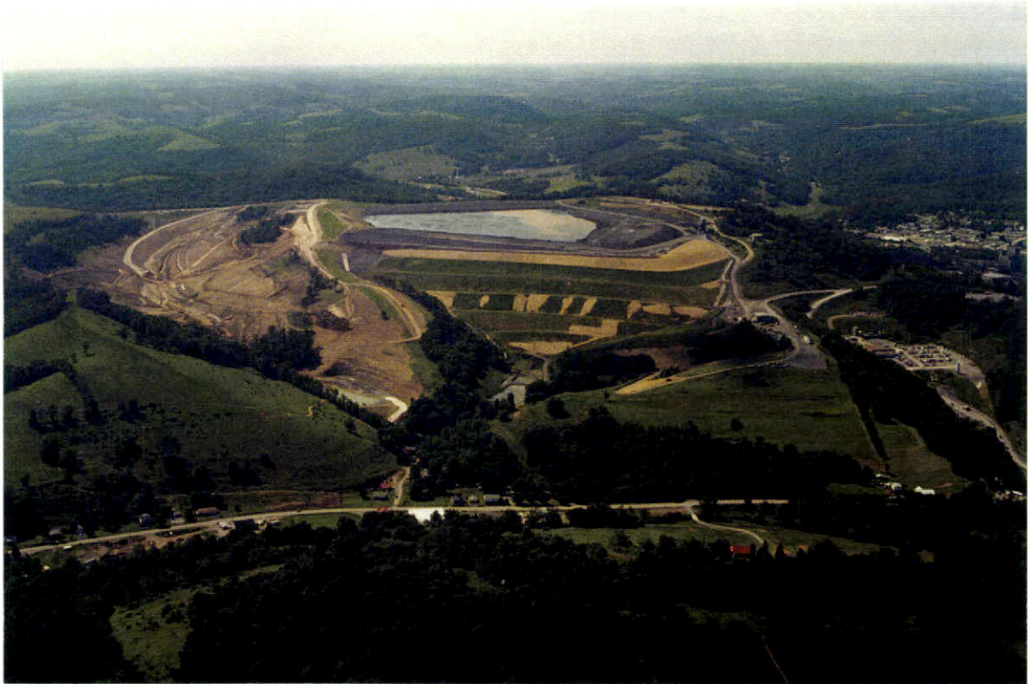
Figure 22. Immense valley fill/slurry impoundment to accommodate longwall mine waste at Waynesburg, Greene County.
