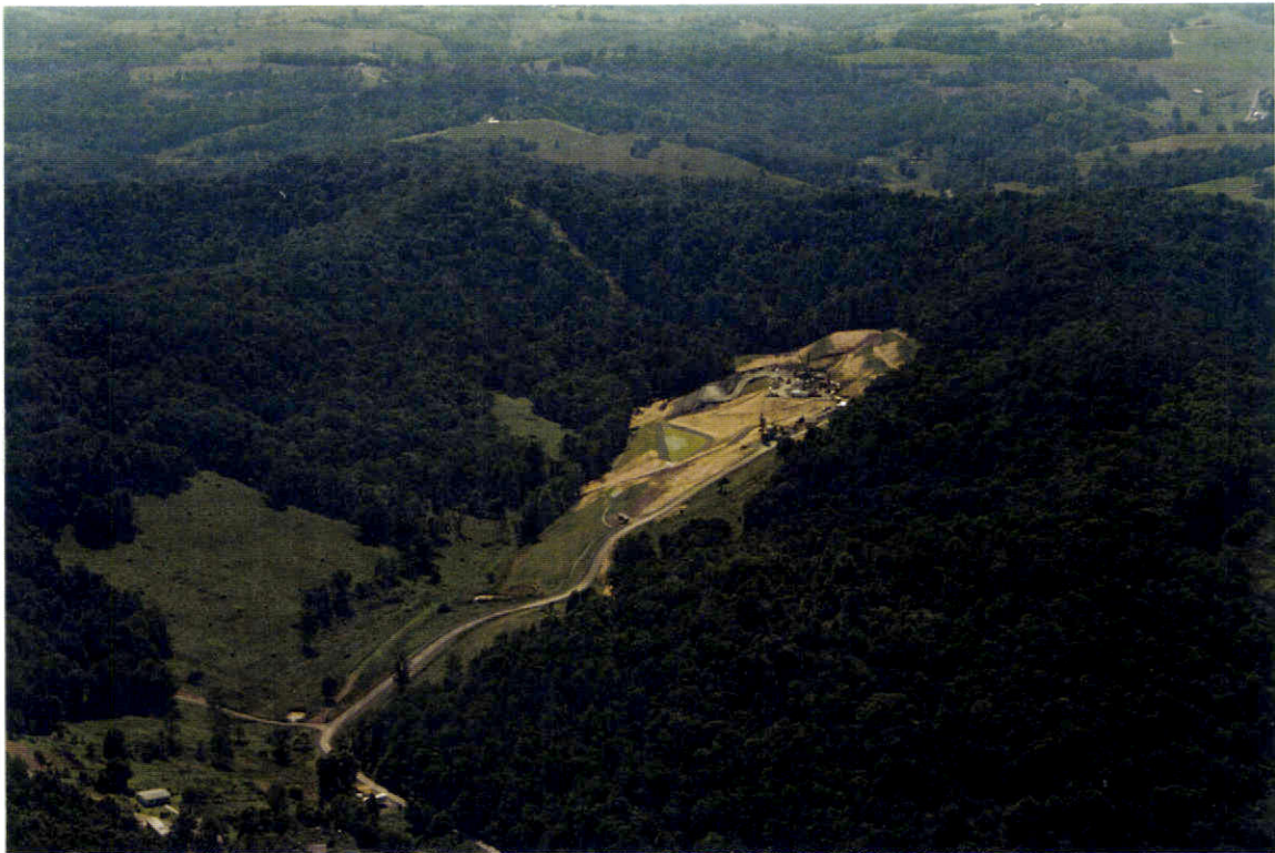
Figure 30. Longwall mine portal, Greene County.
